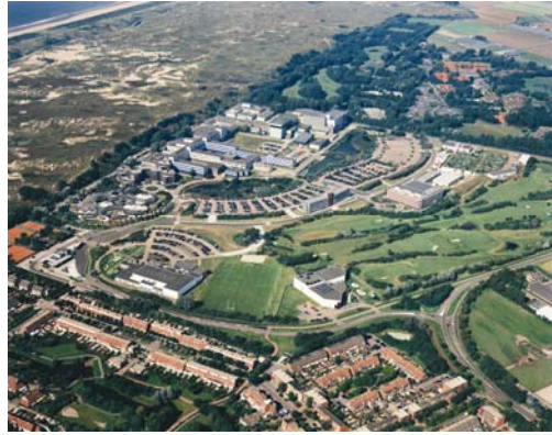
Fig. 1. Aerial view of ESTEC
